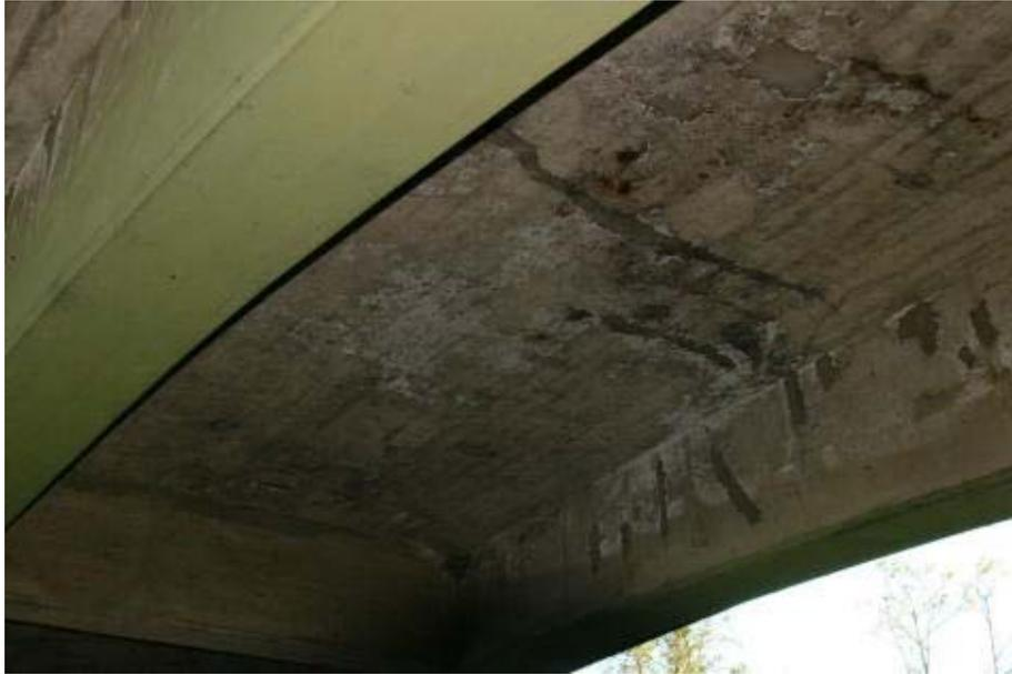
*Photo 3: Cracks and leaching*
