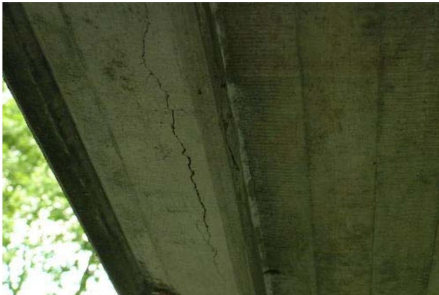
*Photo 2: Cracks in the edge beam*
