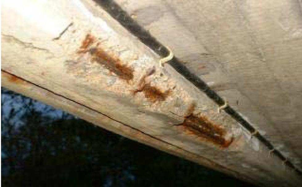
*Photo 1: Corrosion of the reinforcement*
